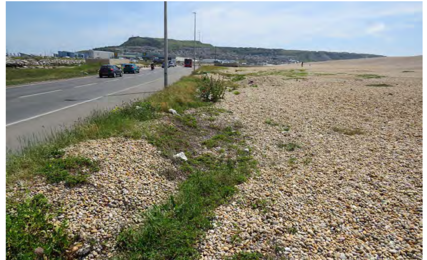
Photo 18: Raised bank formed alongside footway north of Osprey Quay.
